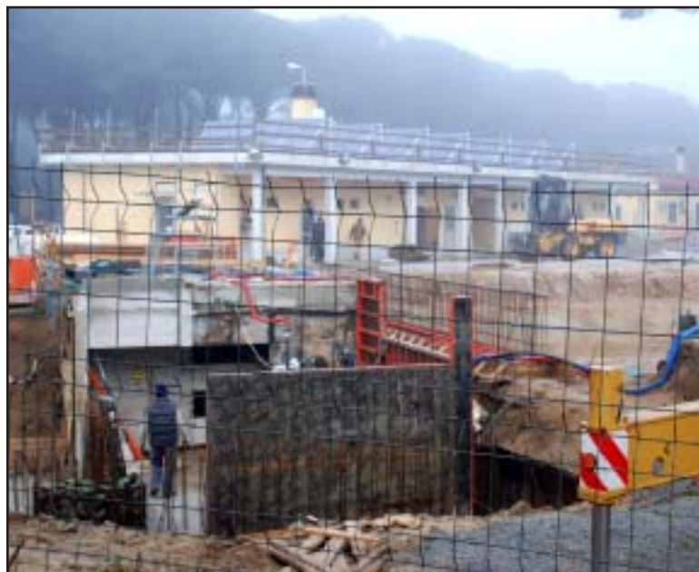
Construction workers in the shell of new Camp Darby pool.
